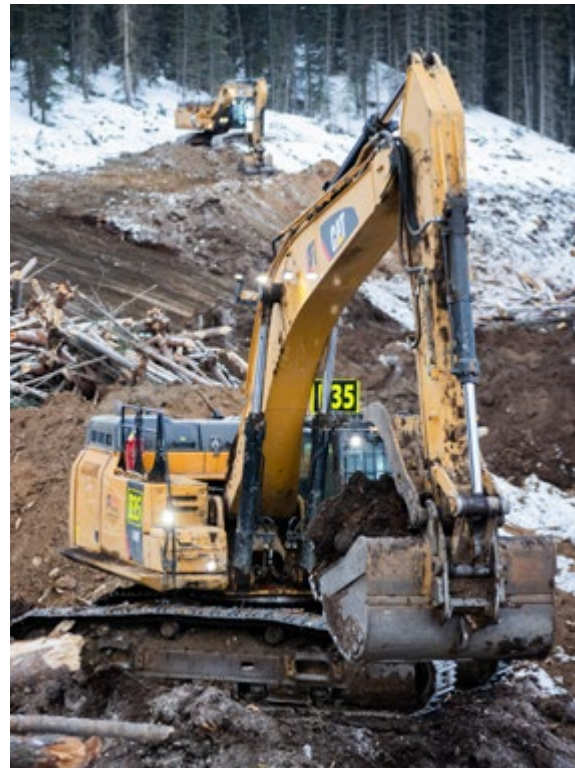
Above: A TNDC excavator at work at Red Chris.
