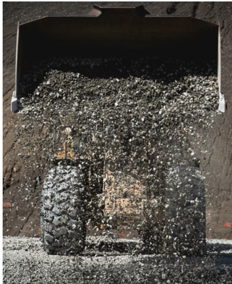
Left: Gravel being laid in construction of the Red Chris TIA.
